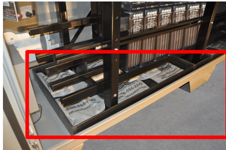
Battery Spill Containment. (n.d.). Retrieved June 07, 2019, from https://www.sbsbattery.com/products-services/by-product/battery-spill-containment-systems.html
